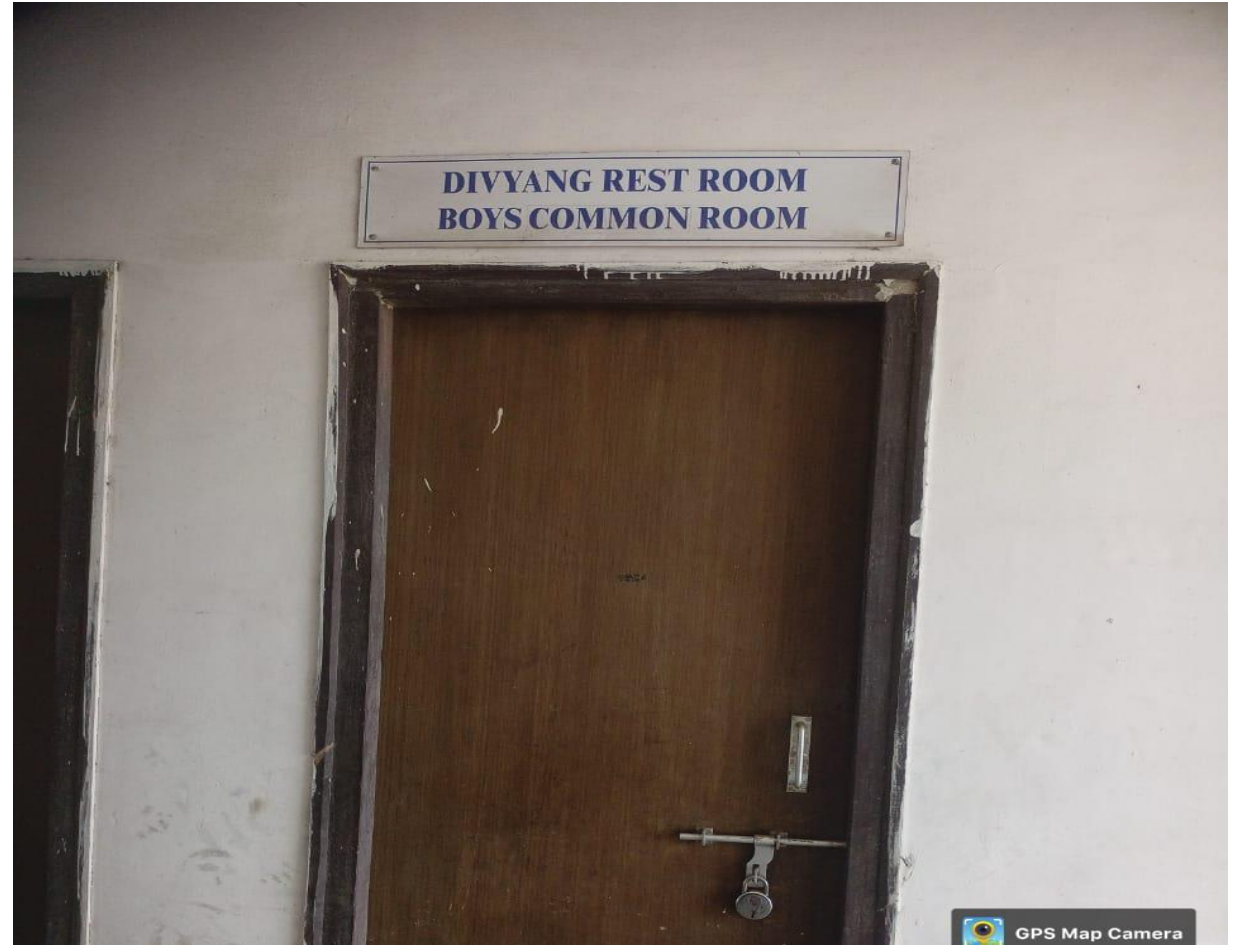
Divyang Rest Room Boys Common Room
